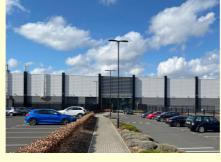
Built and accredited to Uptime Institute Tier 3 specifications, the secure and resilient 63,055ft<sup>2</sup> facility has capacity for up to 2,000 racks in three separate data halls. There is currently 6MW of IT power available, with the potential to increase this
